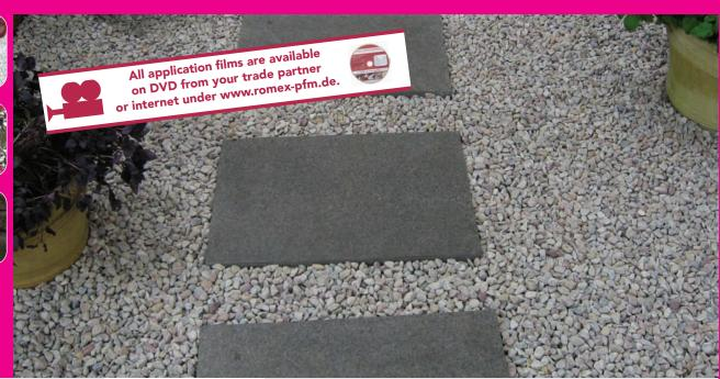
ROMPOX® - DEKO is a binding agent for the hardening of commercially available washed, dried and dust-free grit and gravel (granularity of approx. 5/8 to 32/56 mm) in- and outside. Kindly note the following examples:
